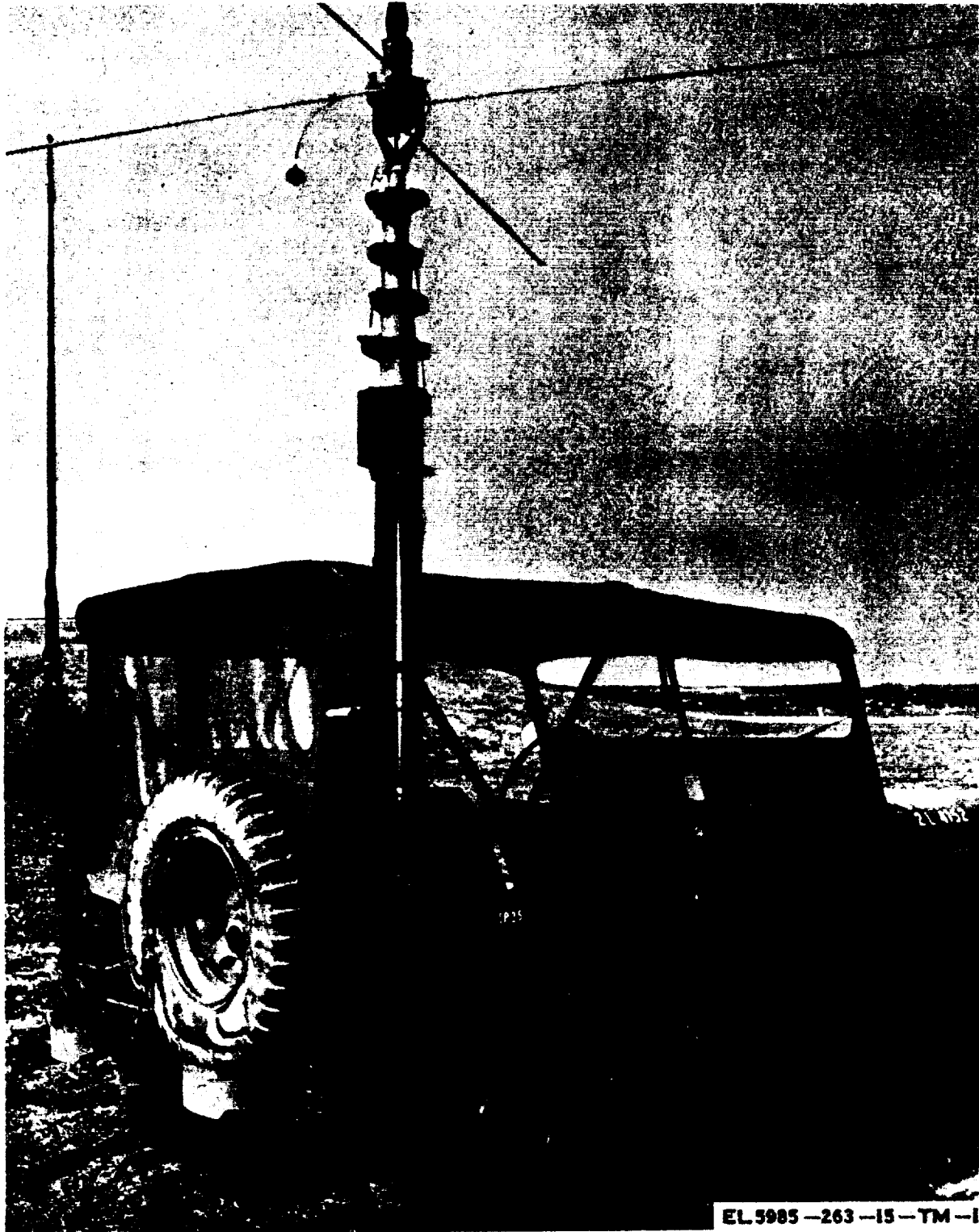
Figure 1-2. Typical vehicular installation of Mast AB-903/G.
